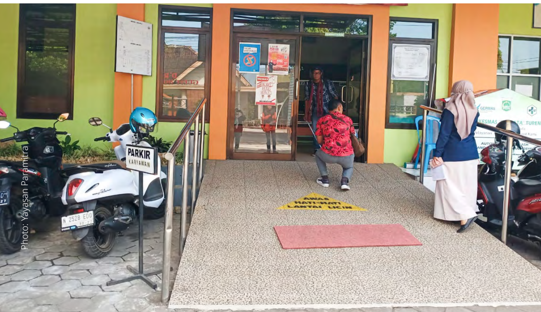
Puskesmas in Turen, one of MADANI's pilot locations in Malang district, has upgraded the entrance with a ramp to improve access for people with disabilities, among others, as a way to provide better health services for visitors by applying minimum service standards.
